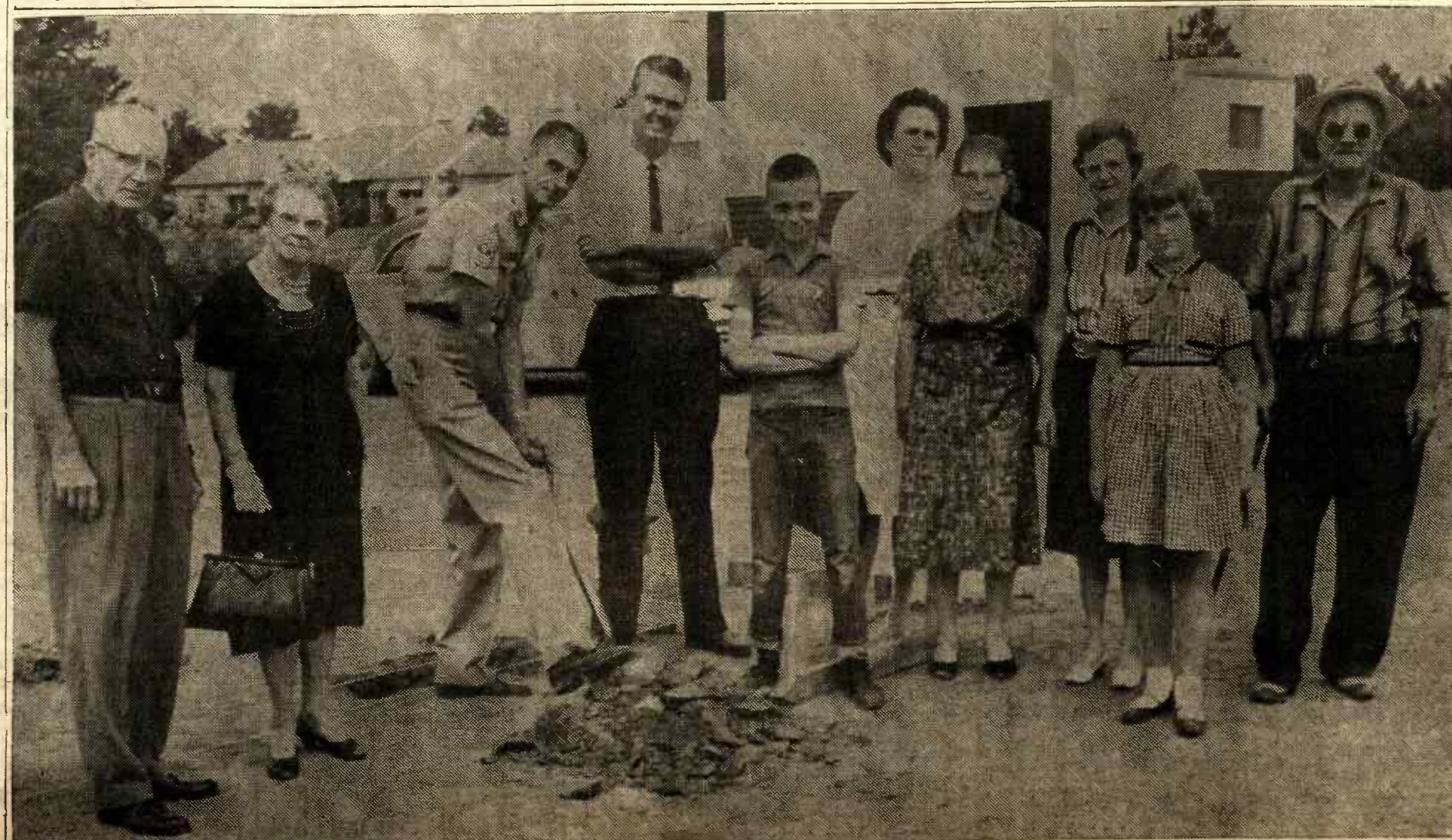
GROUND BREAKING CEREMONIES—Were held Tuesday, August 13, for the Iuka Church of Christ new building being erected on Hwy. 25 South. Members of the congregation present for the event were: left to right, J. W. Ho-
